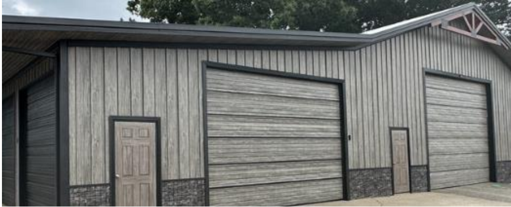
Board and Batten look metal siding with faux stone look vinyl wainscoting.
